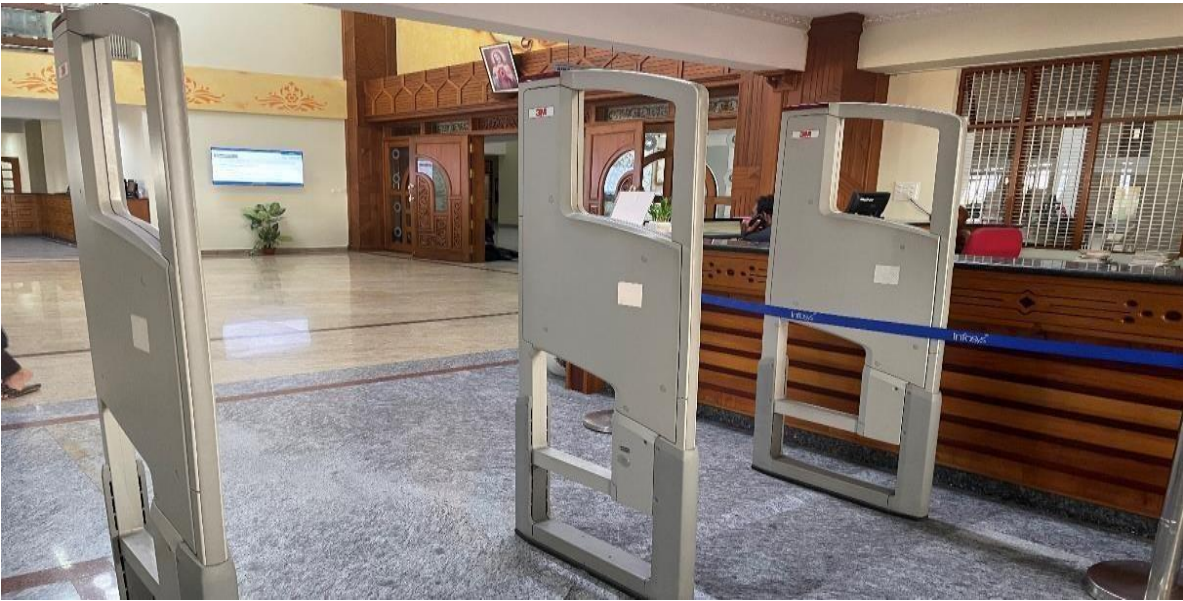
3M Anti-theft Gates installed at the 'Exit'
